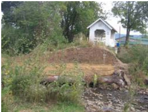
Bank stabilized with wood and vegetation
