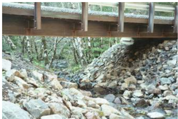
New bridge over stream with Wiley Creek visible in background
