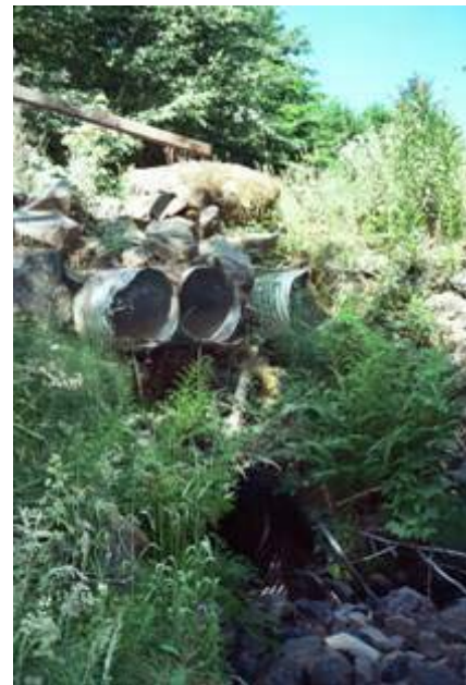
Culvert on tributary to Wiley Creek
