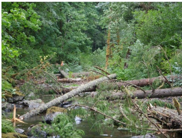
Placing logs with helicopter, August 2008
